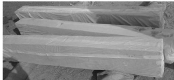
*FIG. 3. BEAMS COVERED WITH PLASTIC SHEET BEFORE BAKING*
