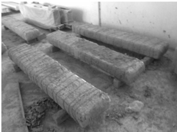
*FIG. 6. A LAYER OF MUD AND CHAFF APPLIED TO CLAY BEAM*
