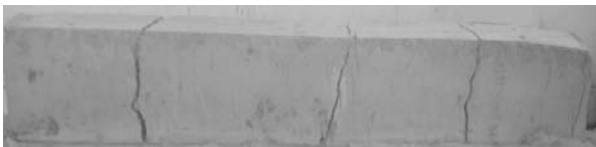
FIG. 5. DRYING CRACKS IN CLAY BEAM
