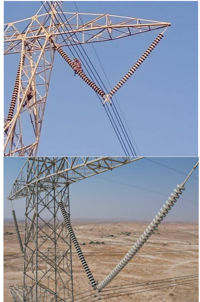
Fig. 2. Conventional Manpower Based Insulator Inspection Methods.
