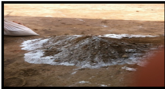
Fig. 5: Mixing mechanism of brick sample preparations
