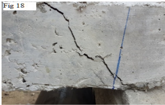
Fig. 18: Failure of control slab S1 in Flexure
