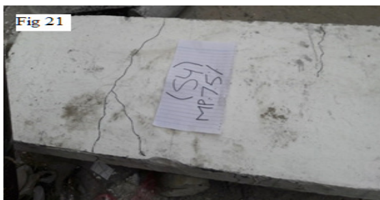
Fig. 21: Failure of Slab S4 (7.5%) in Flexure and Shear
