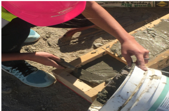
Fig. 8: Mixing the concrete and pouring it into the mold
