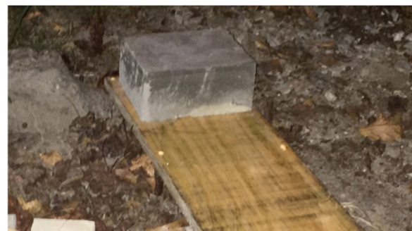
Fig. 11: The forms were removed, leaving four equal sized concrete blocks
