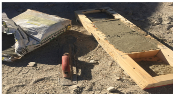
Fig. 9: All the compartments were filled to the top and levelled
