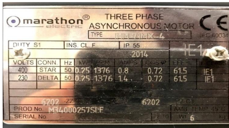
FIG. 24. NAME PLATE DATA OF INDUCTION MOTOR
