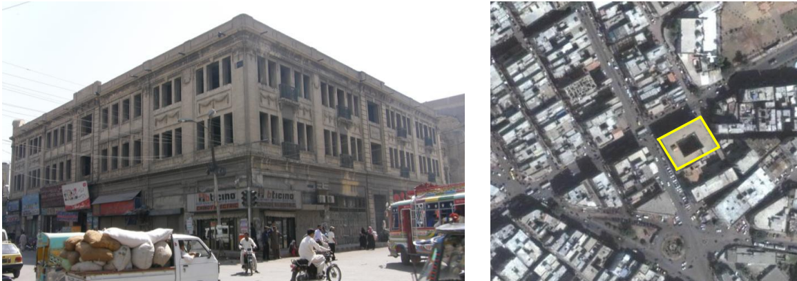
FIG. 6. LEFT – VIEW OF SEVAKUNJ HOSTEL FROM THE CORNER RIGHT – LOCATION MAP OF SEVAKUNJ HOSTEL NEAR PAKISTAN CHOWK
