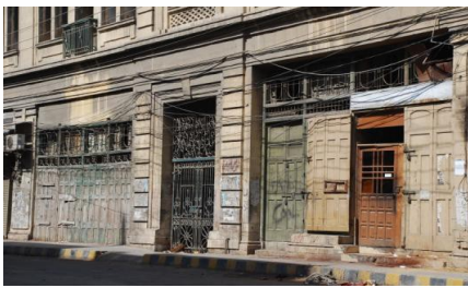
Ground Floor converted into shops
