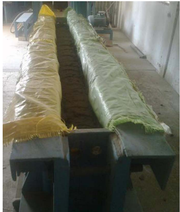
FIG. 1. WALL UNIT BEING CAST IN MOULD
