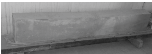
FIG. 7. CLAY BEAM WITHOUT ANY SHRINKAGE CRACKS
