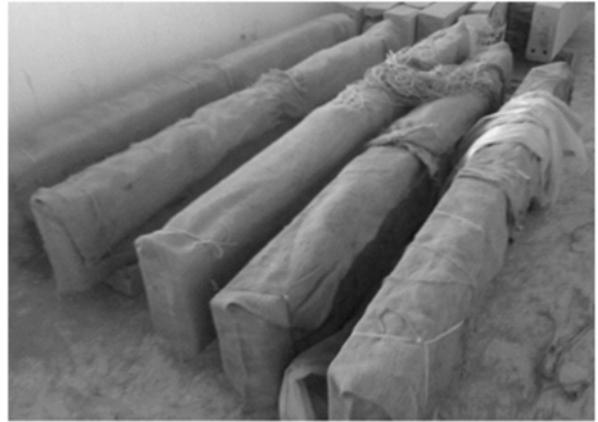
*FIG. 7. BEAMS COVERED WITH GUNNY BAGS*
